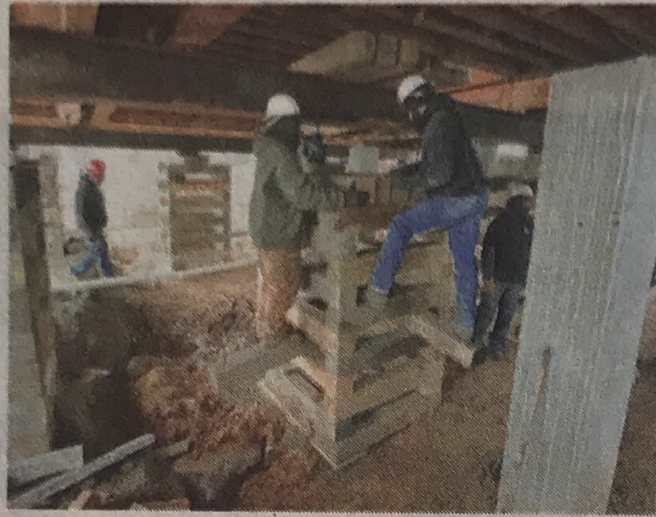
The underside view of the house.
